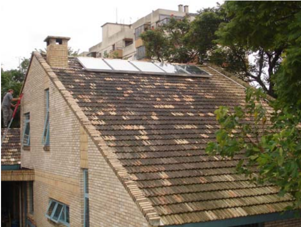
Picture 8.2.3: Installation of solar water heaters in Porto Alegre
